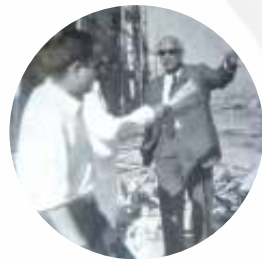
Dissolving Wood Pulp & VSF plants at Harihar, Karnataka commissioned based on in-house engineering
