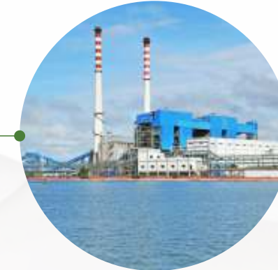
New state-of-the-art VSF plant commissioned at Vilayat, Gujarat
